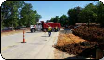
Filling excavated road widening section with recycled ABC from RDU
